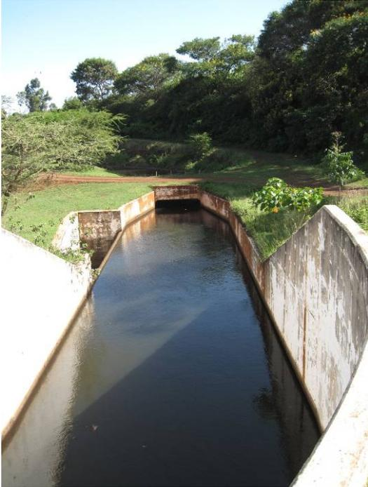
The scheme is served by the Nyamindi and Thiba rivers. From these irrigation water is abstracted by fixed intake weirs and conveyed and distributed by gravity via unlined open channels. A link canal joins the two rivers, it transfers water from Nyamindi to Thiba River serving about 80% of the scheme.
