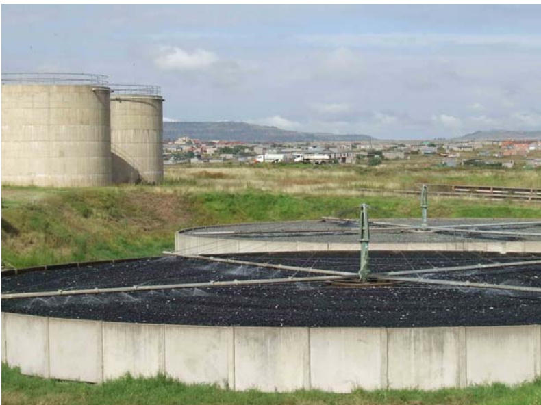
Existing Ratjomose WWTP – trickling filters and sludge digesters
