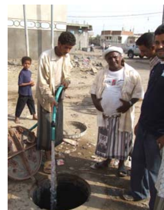
Flushing of sewer in Bait el-Faqih
