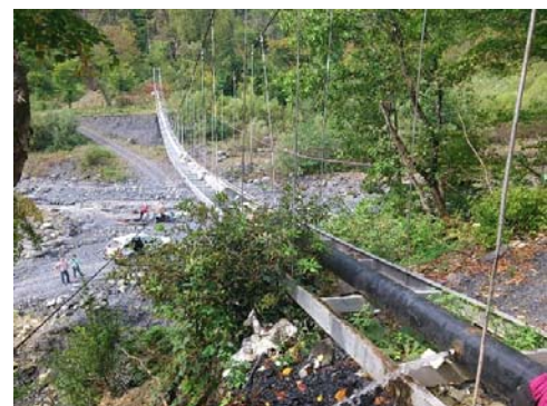
Kvareli Nakhechiskhevi Pipe Bridge
