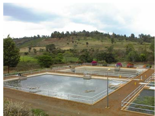
Nyeri STP, sludge digestion lagoons Nos. 3 and 4
